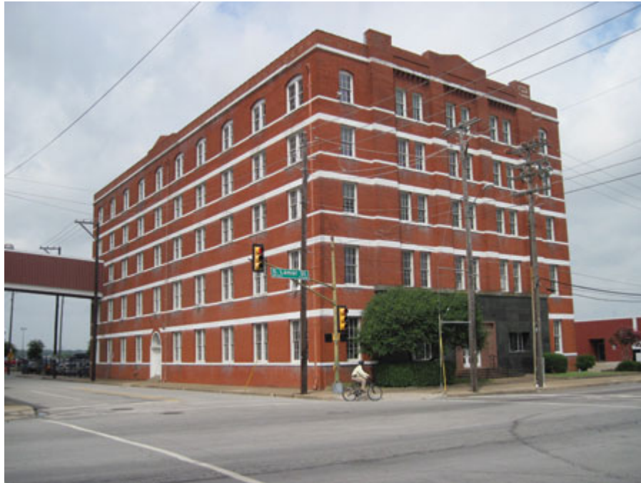
Dallas Coffin Factory Building prior to conversion to Nylo South Side, looking northwest.
