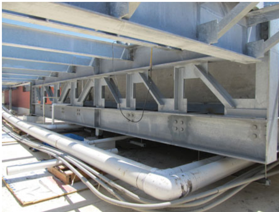
Cantilevered galvanized steel truss on east side of pool, looking southwest.
